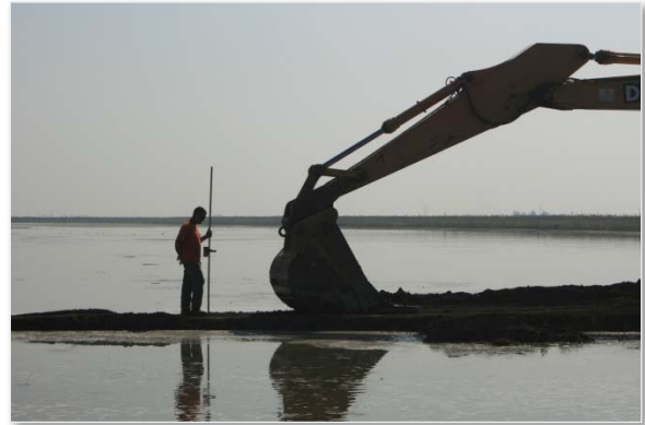
Off-site restoration and mitigation bank construction at the Shin Kee project in Lodi, California
