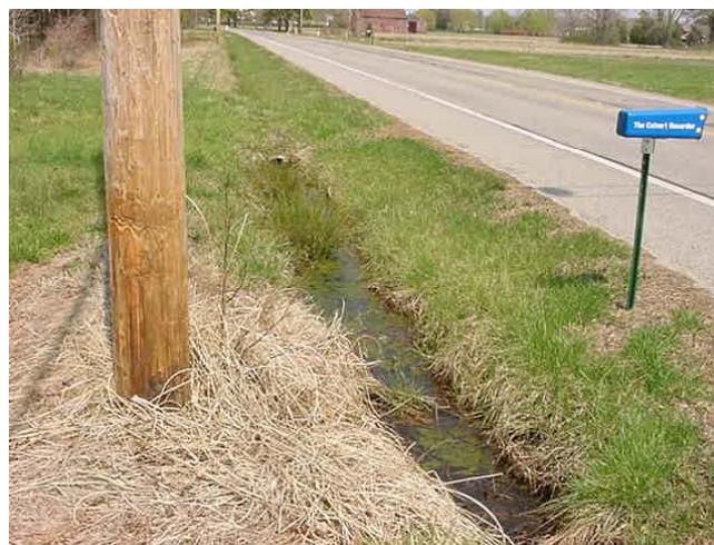
Roadside ditch with ordinary high water mark (OHWM); these were typically disclaimed before SWANNC but they're often jurisdictional today.
