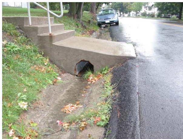
Roadside ditch without OHWM – may not jurisdictional but can serve as a conduit for jurisdiction.
